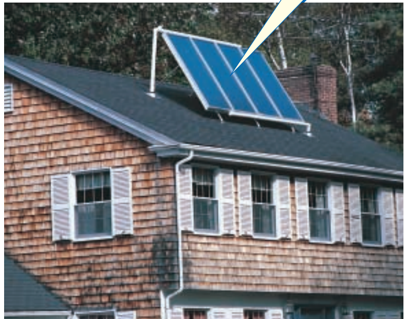
Figure 16 In an active solar heating system, solar energy is absorbed and can be used to heat different rooms in the house.
