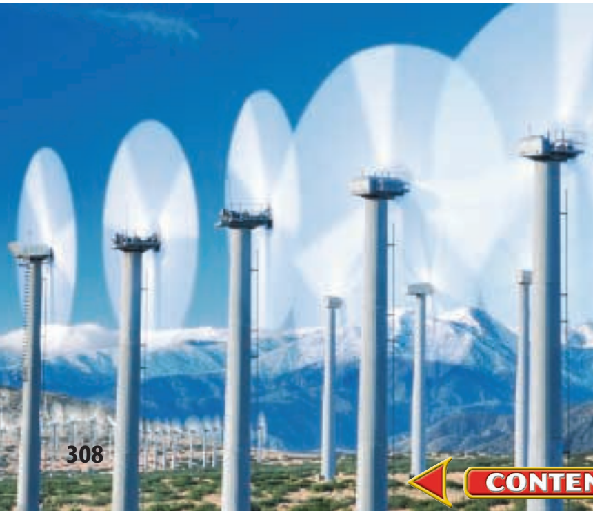
Figure 24 Wind energy is converted to electricity as the spinning propeller turns a generator.
