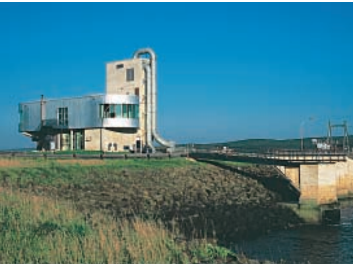
Figure 23 This tidal energy plant at Annapolis Royal, Nova Scotia, generates 20 megawatts of electric power.
