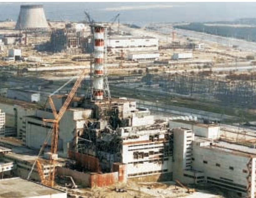
Figure 16 An explosion occurred at the Chernobyl reactor in the Ukraine after graphite control rods caught fire. The explosion shattered the reactor's roof.
